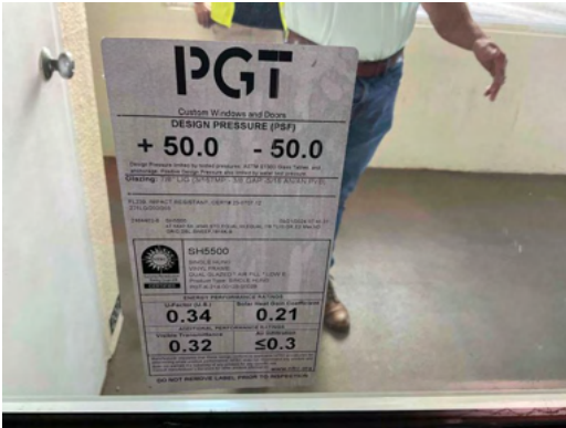
Photo 15 Unit No. 202 - View of PGT Design Pressure Sticker on New Window.
