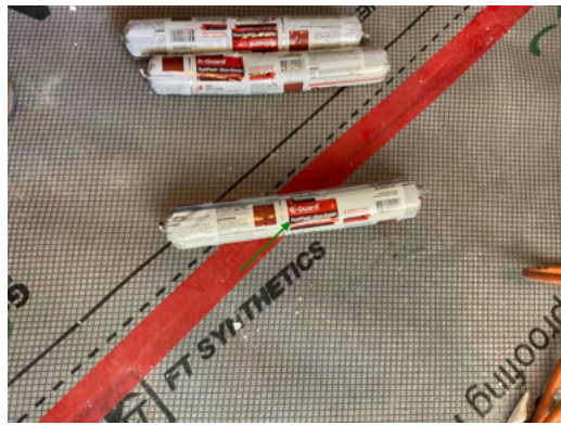
Photo 8 Unit No. 1112 - View of materials on site.
