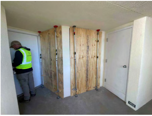
Photo 7 Unit No. 1102 - View of exterior protection installed at window replacement location.
