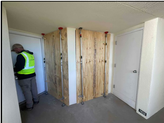
FIGURE 5 - Unit No. 1102 - View of exterior protection installed at window replacement location.
