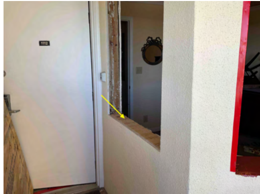
Photo 10 Unit No. 1112 - View of existing window removed - Work in progress.
