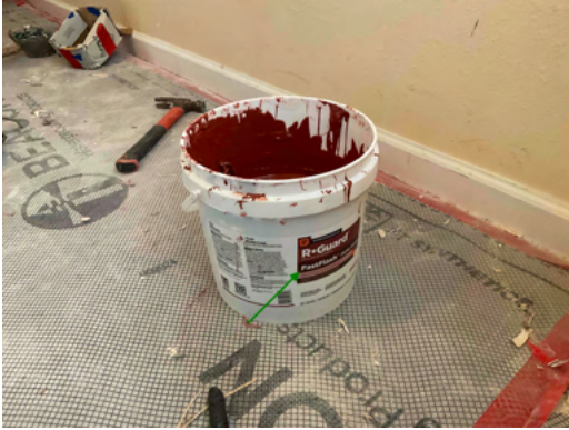
Photo 9 Unit No. 1112 - View of materials on site.
