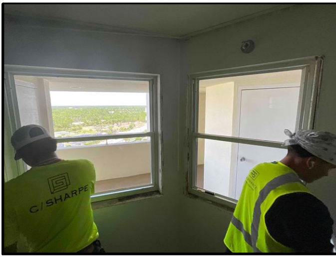
FIGURE 3 - Unit No. 1104 - View of existing windows being removed for replacement.
