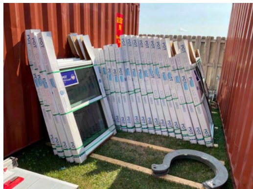
Photo 24 Materials On-Site - View of approved PGT SH5500 Windows stored for window replacement.
