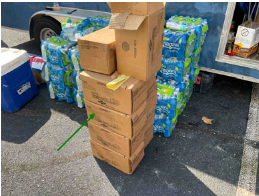
Photo 23 Materials On-Site - View of approved DowSil 790 silicone sealant stored.
