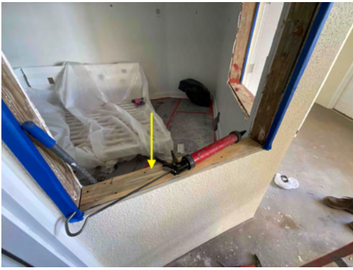
Photo 7 Unit No. 1102 - View of existing window removed - Work in progress.
