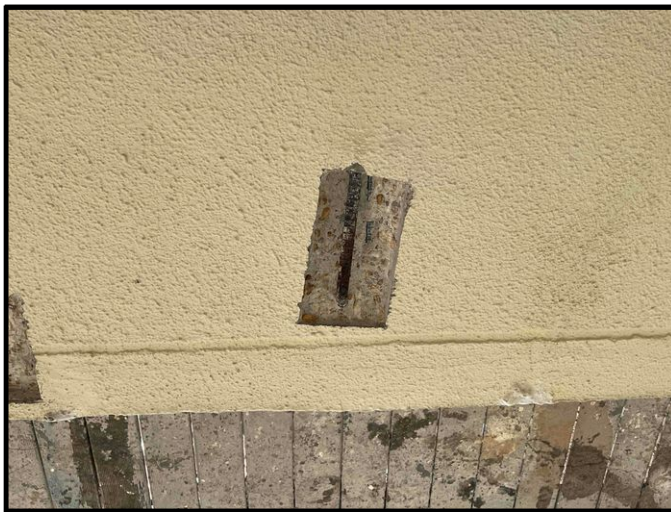
FIGURE 9 - Unit No. 912 - View of partial depth repair mock-up in progress.
