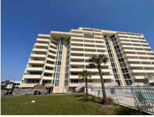
Photo 1 South Elevation - Overall view.
