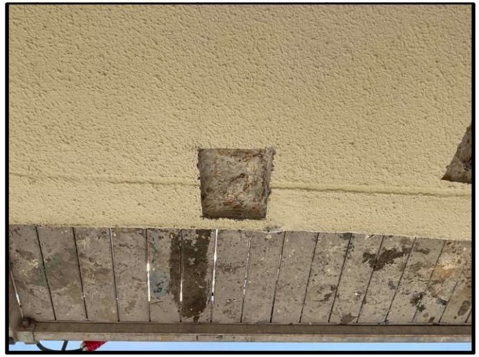
FIGURE 8 - Unit No. 912 - View of rod chair repair mock-up in progress.
