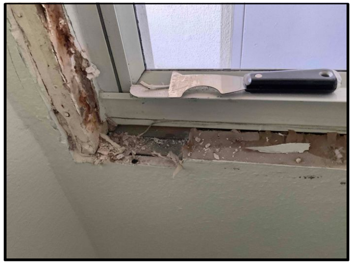
FIGURE 4 - Unit No. 1104 - View of existing windows being removed for replacement.
